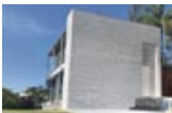
Elementi prefabbricati e in calcestruzzo, Coudrey house, Australia
